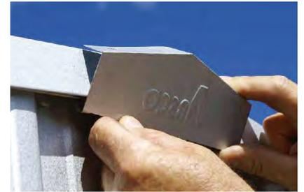
Bend the top and bottom flanges as shown, then hook the bottom flanges under the top channel and screw top to the ridge beam with two screws.
