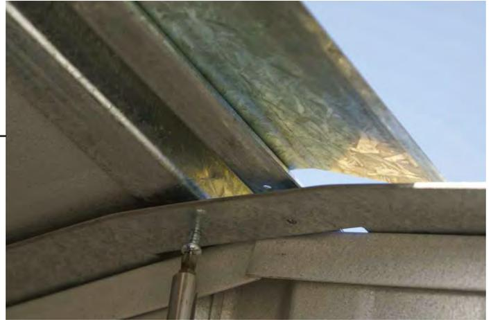
Secure peak brace to ridge beam and roof panel with one screw at each end
